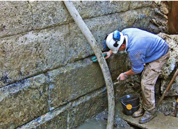
Roman quay wall at Marseille (France) built with ashlar stretchers (Inrap, 2006)
