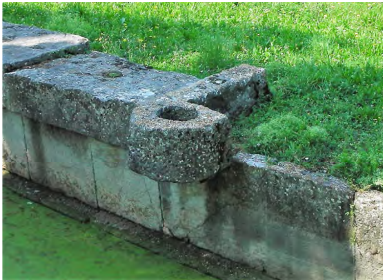
Possible foot-hole of a derrick mast at Aquileia (Italy), (Photo de Graauw, 2010)
