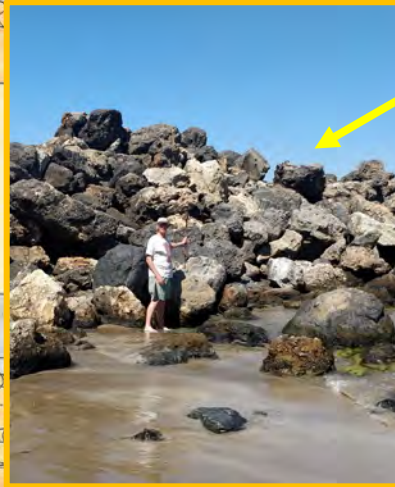
Rubble-mound breakwater at Kissamos (Crete) (Photo de Graauw, 2022)
