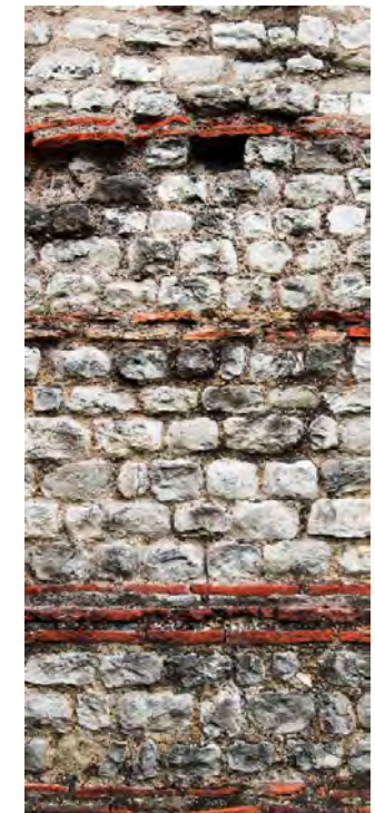
Courses of bonding tiles in the London Wall
