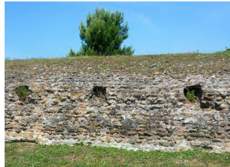
Portus' north concrete breakwater showing imprints of transverse caisson beams (Photo de Graauw, 2011)
